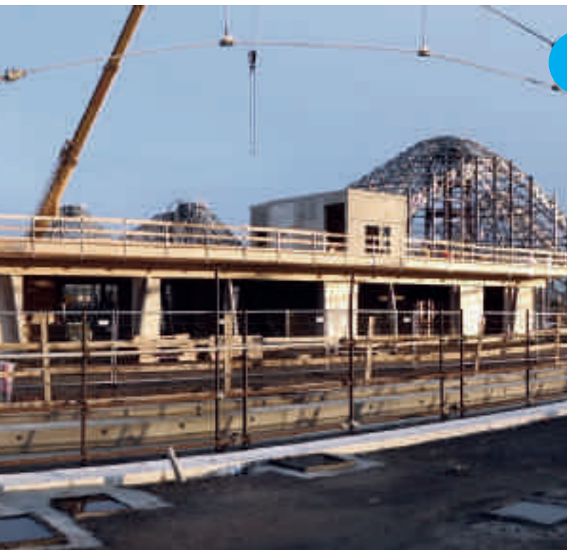
Stratex solves complex and demanding construction tasks related to the Expo 2015 in Milan. As their partner, Hilti provides comprehensive on-site solutions and services.
