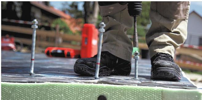
The HCW and HCW-L feature an integrated clamping mechanism for easy push-to-fit installation with Hilti anchor systems.
